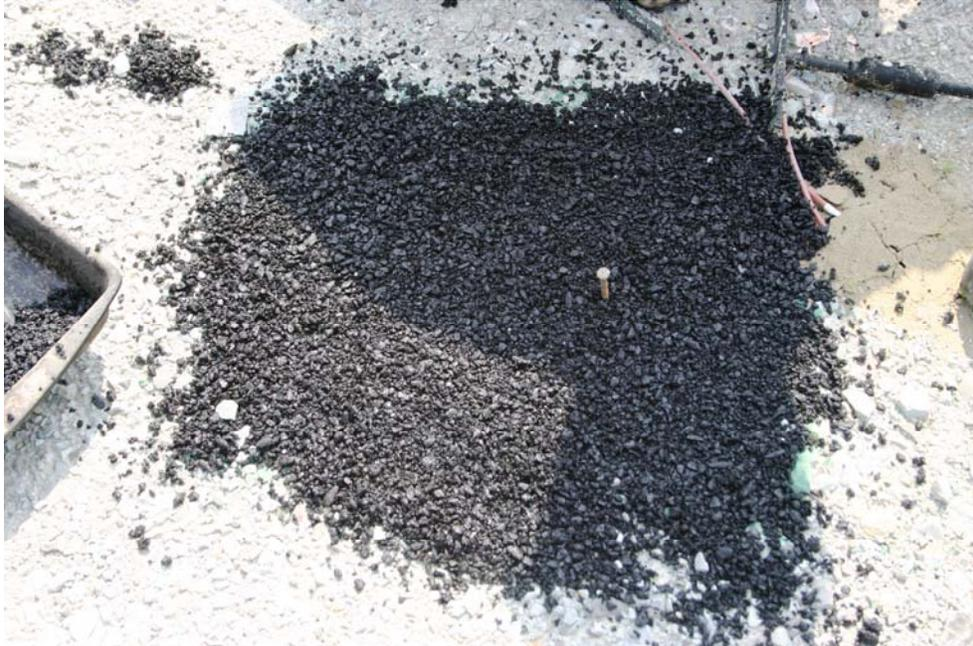
**Figure 4.9 – Bottom Asphalt Cushion and Alignment Nail**
