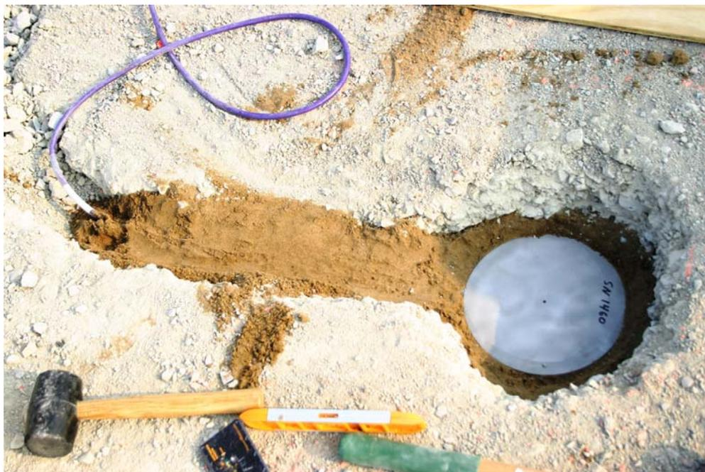
**Figure 4.5 – Installed Base Course Earth Pressure Cell**
