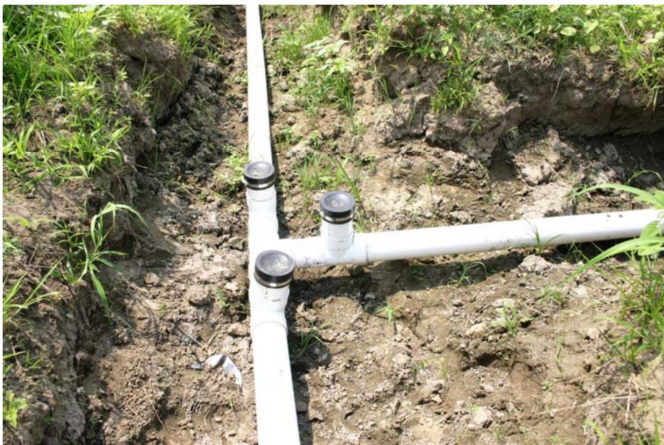
**Figure 5.9 – Junction Located at the Base of the Lateral**
