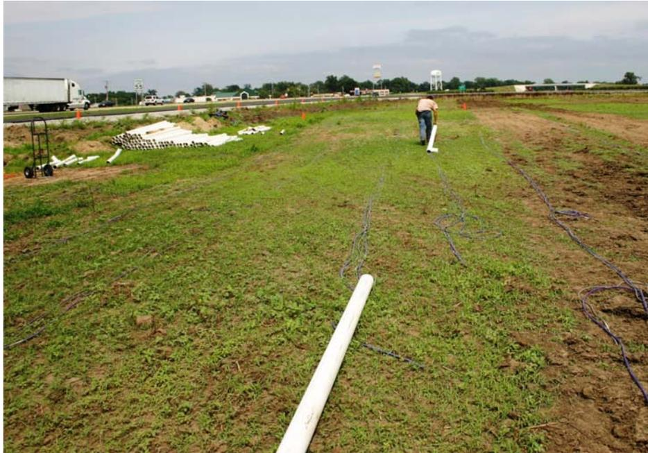
**Figure 5.10 – Pipe Feeding Process**
