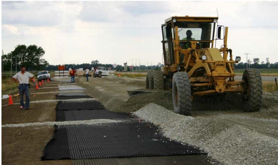
**Figure 5.4 – Aggregate Placement**
