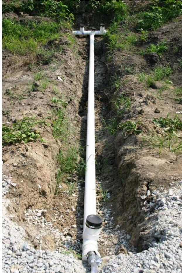
**Figure 5.8 – Lateral Pipe Extending From the Shoulder to the Header**
