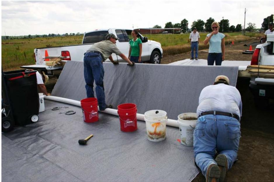
**Figure 5.3 – Geosynthetic Lay Down Technique**
