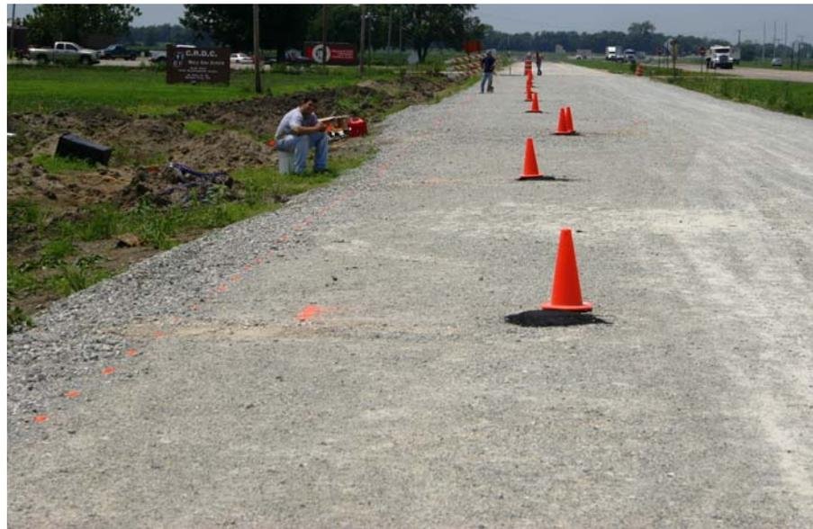
**Figure 5.5 – Final Base Course with Asphalt Strain Gages**
