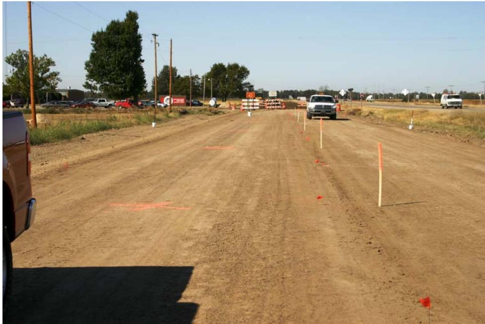
**Figure 5.1 – Finished Subgrade**
