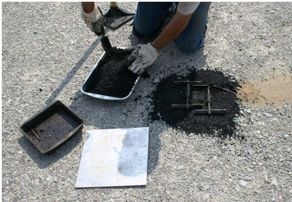
**Figure 4.10 – Strain Gage Installation In Progress**
