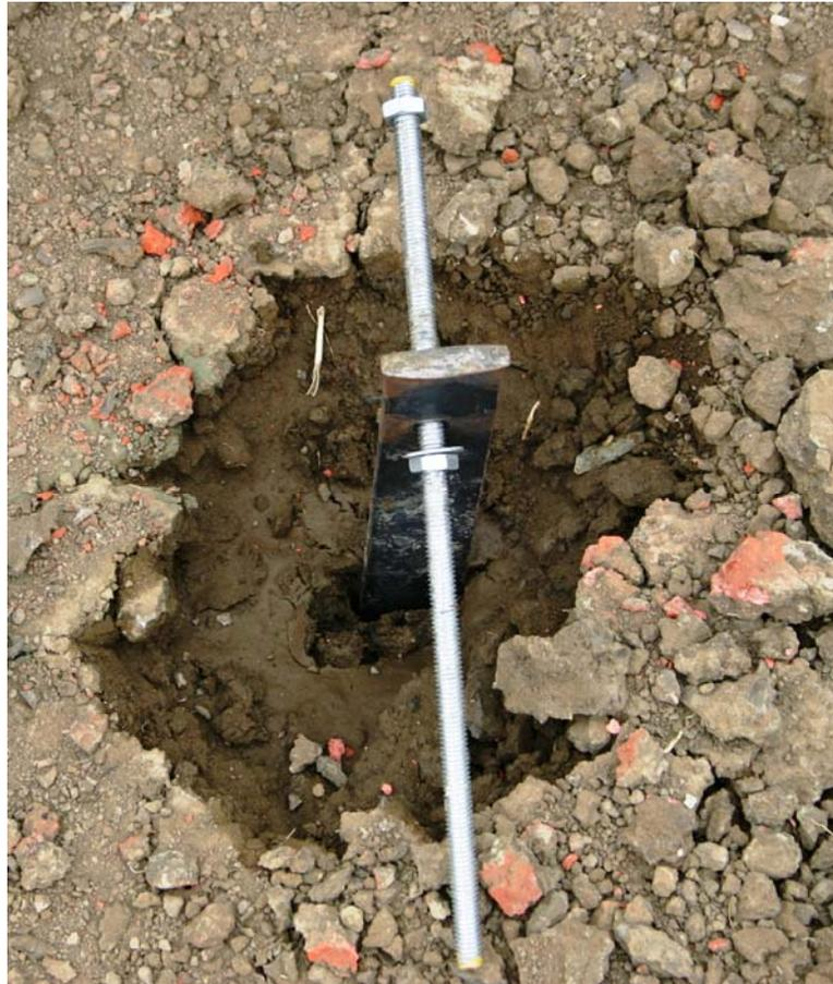
**Figure 4.19 – Insertion of Metal Bar with Leverage Rod**
